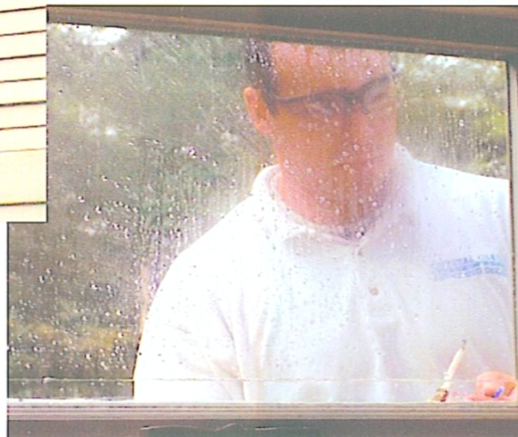
(above and right) The CCWW process begins with an assessment of the IG. The process is designed to remove moisture and fogging from failed IG units.
