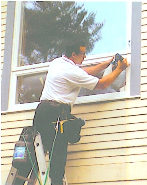
(above and right) The CCWW process begins with an assessment of the IG. The process is designed to remove moisture and fogging from failed IG units.
