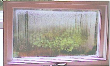
The CCWW process is applied to failed IGU units (right) to remove fogging that may have occurred (above).
